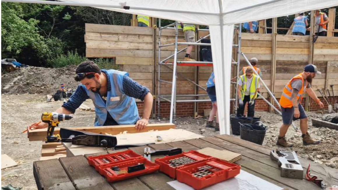
SPAB Fellows working on the Old House project
