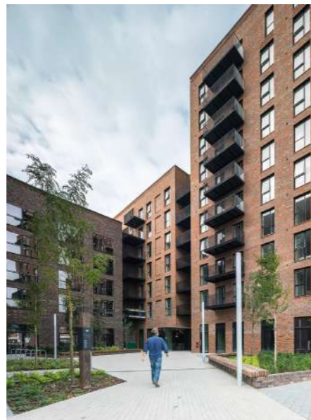
Dalston Lane London - one of the UK's largest timber construction projects. Daniel Shearing courtesy Waugh Thistleton Architects
