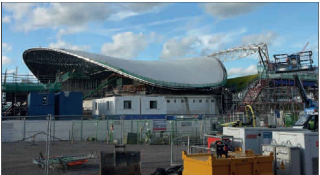
The Aquatic Centre under construction
