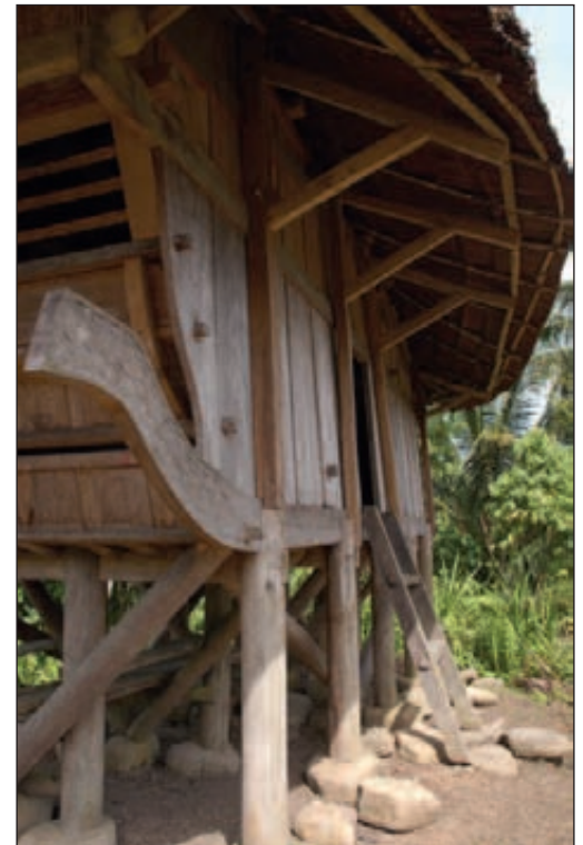
New house built by the Carpentry course
