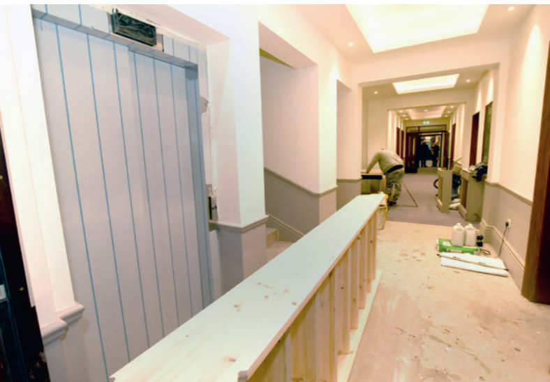
Ongoing work in December
