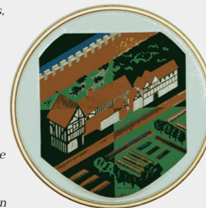
Carpenters' Hall in 1429 (roundel by Jean Clark)
