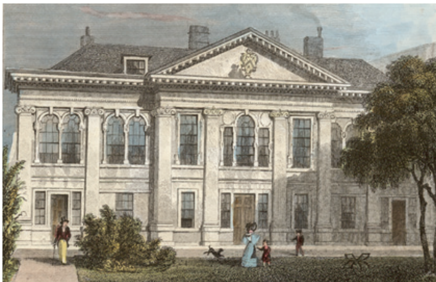
The 1664 West Wing of Carpenters’ Hall as it was in the early 19th century
