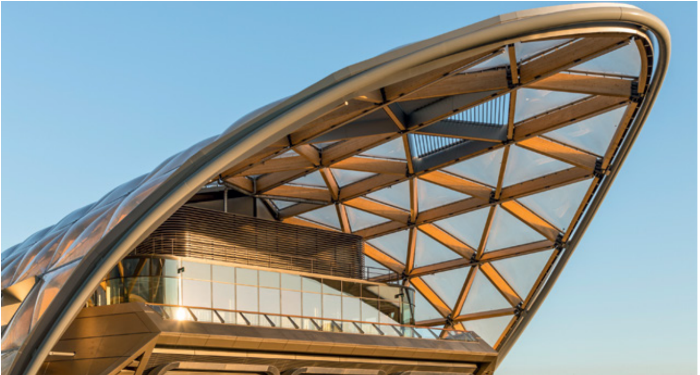
Canary Wharf Crossrail's spruce lattice roof
