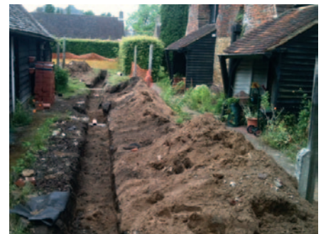
Repair work to the drains at the Almshouses
