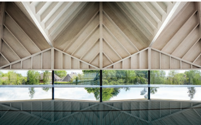
Alfriston School swimming pool's low-level glass strip allows unobstructed views and makes the roof appear to float
