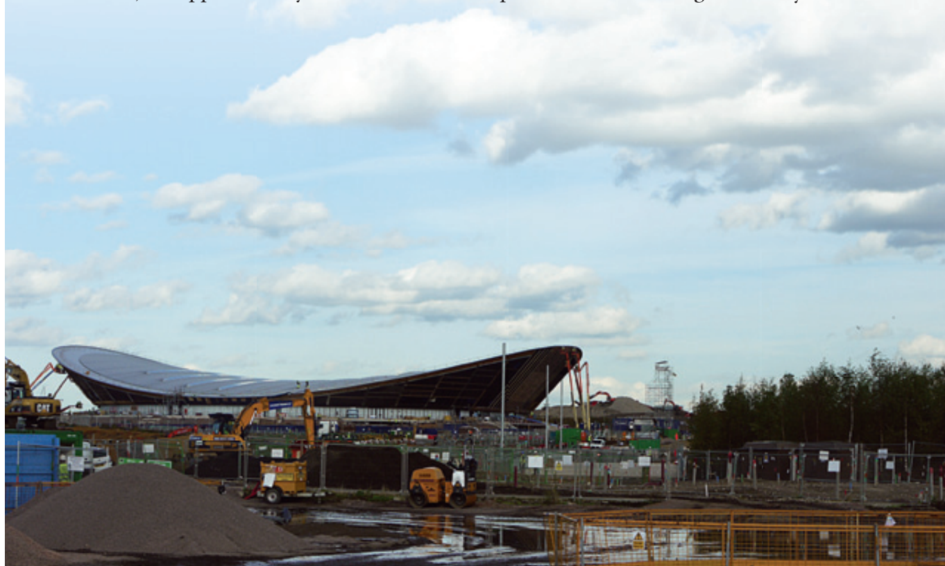
The Olympic Aquatic Centre under construction, 2010
